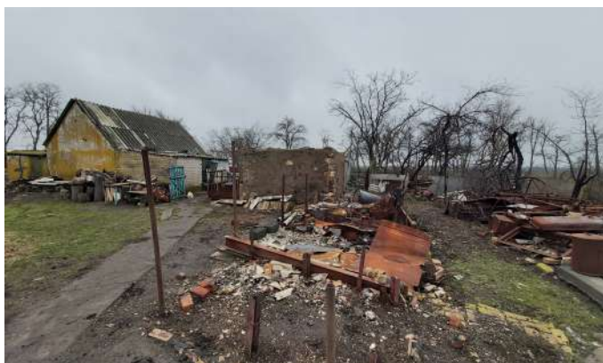
Figure 11 Destroyed housing Khersonska Oblast
