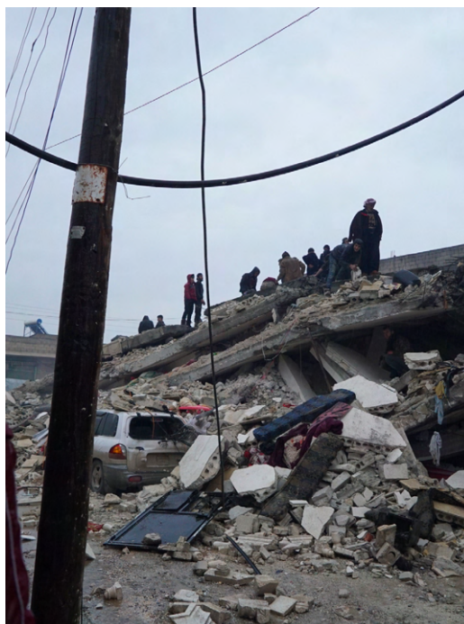
The damage caused by the February 6 earthquake in Jandairis.
